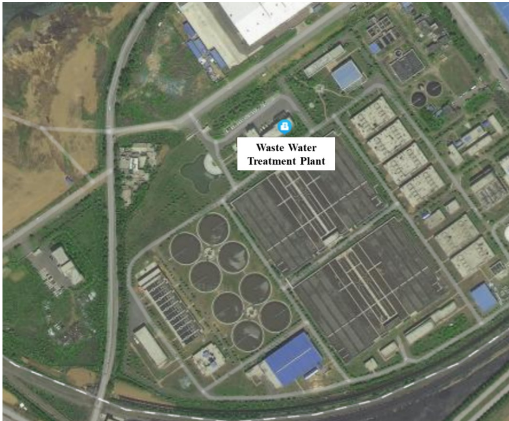
Fig. 1. The satellite image of WWTP structure
